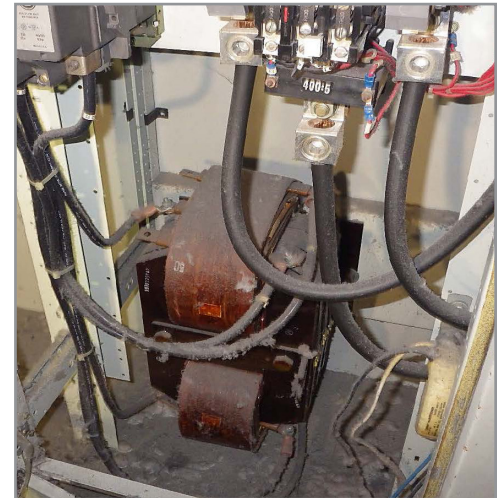
▲ Motor control center (MCC) transformer before decontamination
