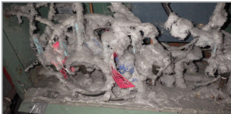
▲ Backside of line R-4 operator's station before decontamination
