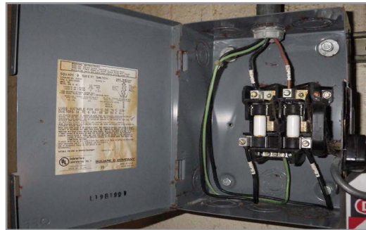
▲ Square D disconnect switch after decontamination
