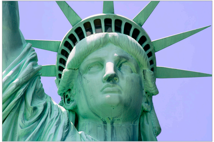
Green patina on the statue due to corrosion
