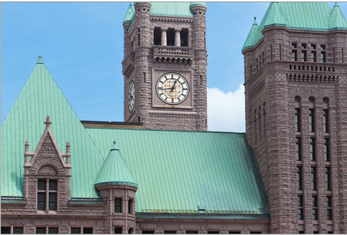
Minneapolis Hennepin county courthouse copper roof
